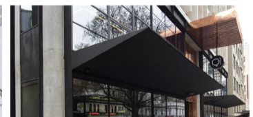
E Dark Painted Steel QT Hotel, Melbourne, Candalepas Associates
