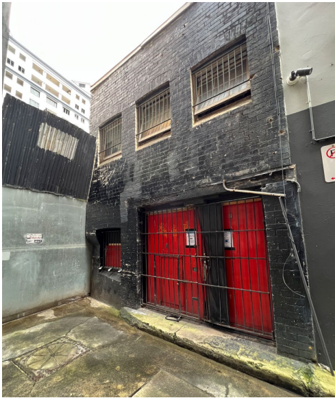
Figure 4-3: Foster Lane access (Source: Curio 2022)
